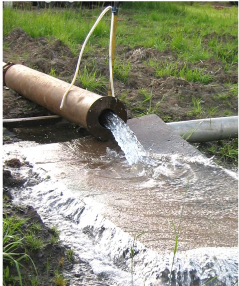
Orifice tube measuring flow from a municipal well
