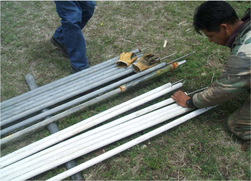
Protect pump and drop pipe from direct contact with the ground during installation and maintenance
