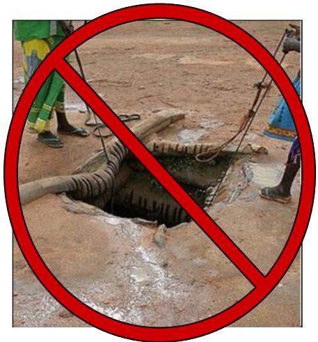
Surface water entering a well.
