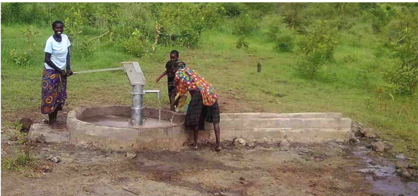
Well head with good apron and drainage
