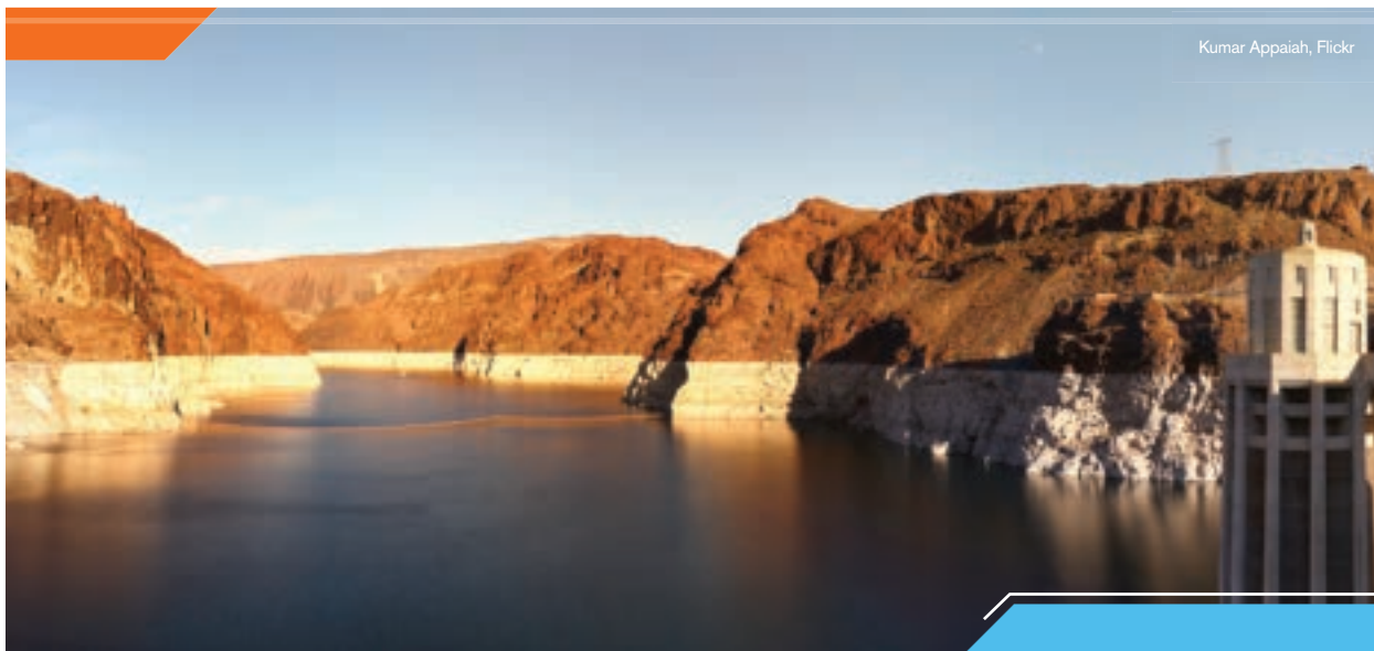
Lake Mead near Hoover Dam, Nevada, USA
